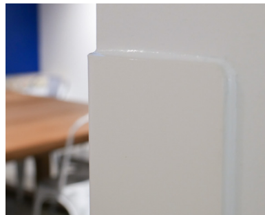
Above: Photo of a completed corner protector installation.
