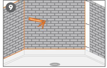
Side wall panels can be installed vertically which will need to be determined prior to the ordering process. This allows full panels to be installed without any seams. This is recommended only if the wall is less than 48"wide. Install adjacent panels as previously instructed. Apply Altro sanitary sealant as shown in drawing at inside corners, as well as top and bottom of all panels to prevent moisture ingress.
