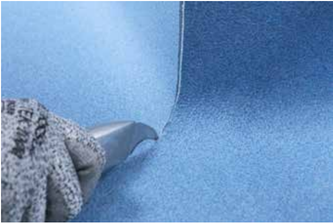
1. Use a concave blade to prepare the upstand and cove former sections, creating a 'V' section in preparation for hot welding.
