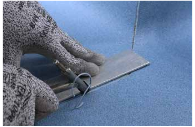
2. Groove the join on the flat section of the floor.
