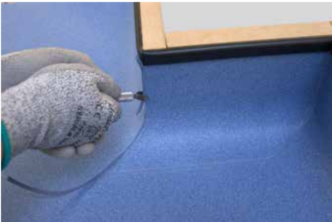
5. Chamfer off the external mitre with the square router blade.
