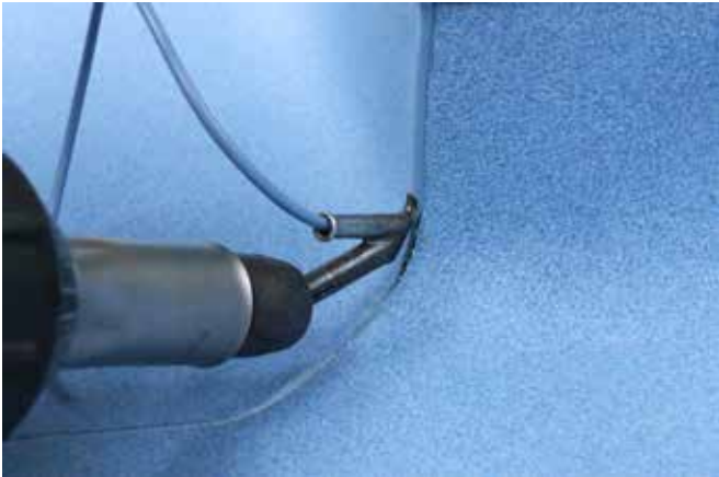
3. Weld the external mitre from top to bottom, being careful not to press the weldrod too firmly on the upstand section as this can cause damage to the flooring.
