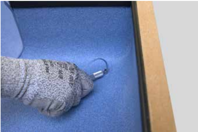
3. Trim the weldrod with the round router blade.
