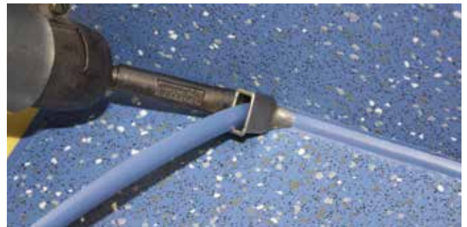
Welding the HB rod
