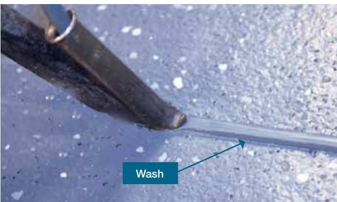
Move heat gun down the seam
