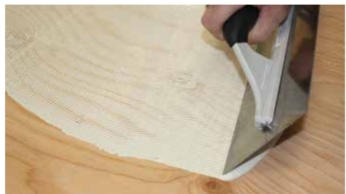
Apply adhesive with appropriate trowel
