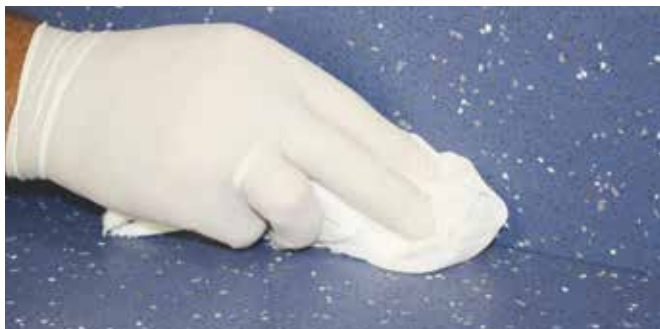
Prep surface with isopropyl alcohol
