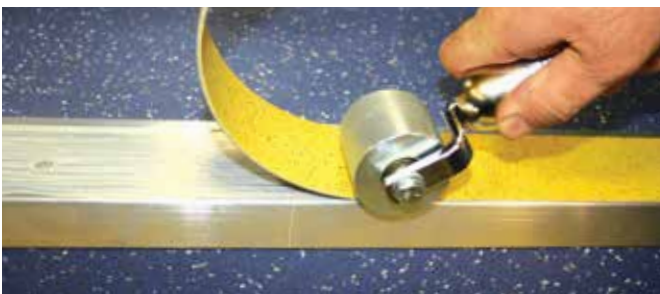
Roll Into place with hand roller
