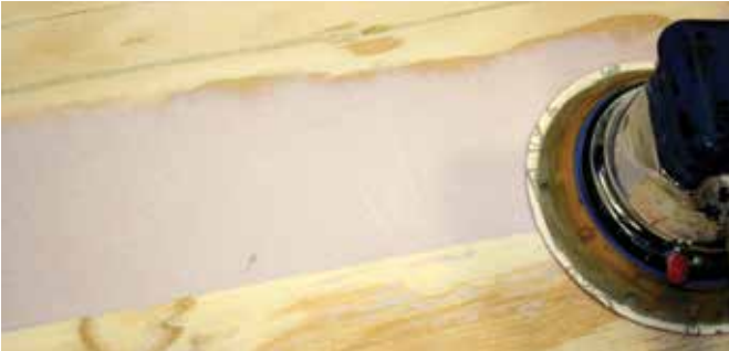
Sand and level the subfloor
