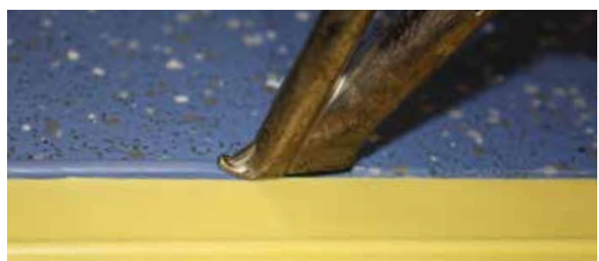
Weld step edge to flooring
