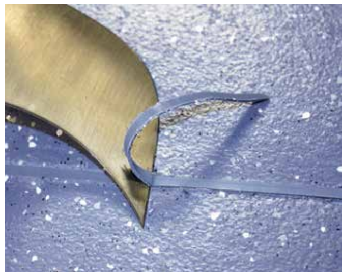
Cut remaining weld with a trim knife
