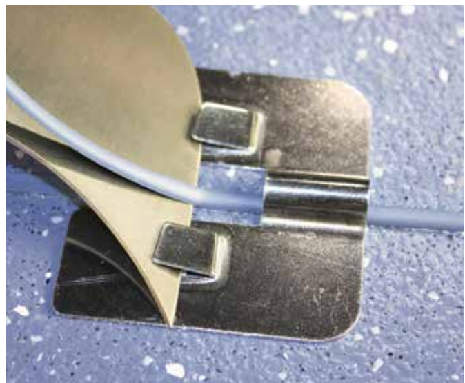
Cut the weldrod with the trim plate
