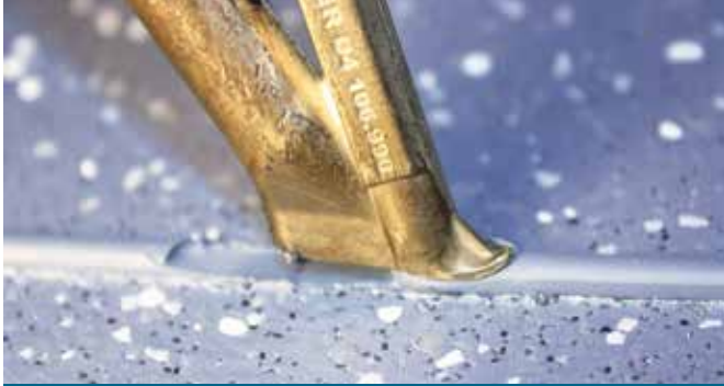
Overlapped weldrod In middle of seam
