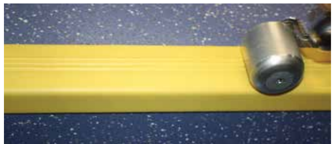
Roll with a hand roller
