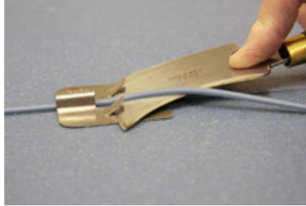
5. Using trim plate and spatula, trim weldrod
