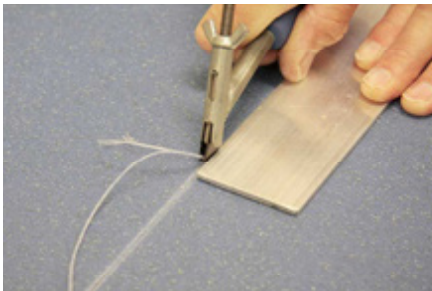
3. Groove to the correct depth
