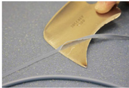
6. Final trim of weldrod using spatula knife
