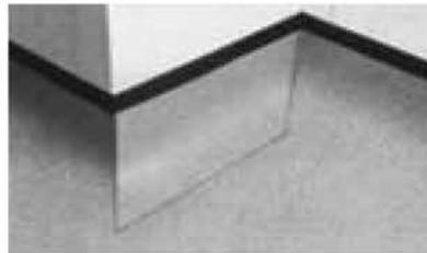
2. Once the main flooring is adhered, cut in the back and front mitres, then cut out the section to remove the make-out.
