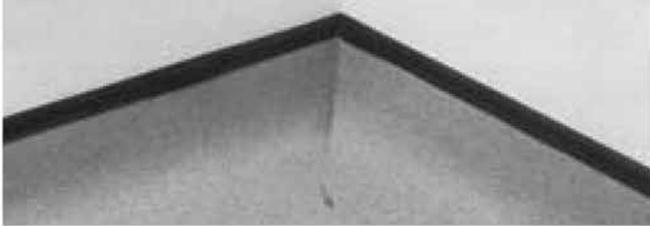
3. Fold in the second side and carefully cut in to complete the joint. Adhere and hot-weld the joint.
