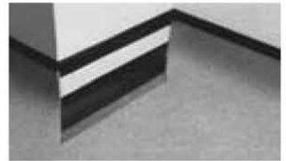
3. Take a separate piece of flooring roughly cut to size, apply adhesive, position and cut to fit the back internal mitre. Cut in the front external mitre. Groove and hot weld to complete the section.
