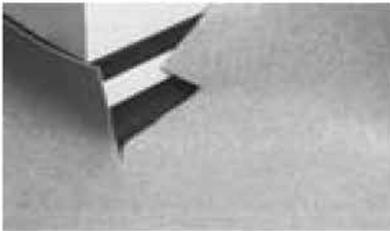
1. Roughly cut the flooring oversize to meet the required section.
