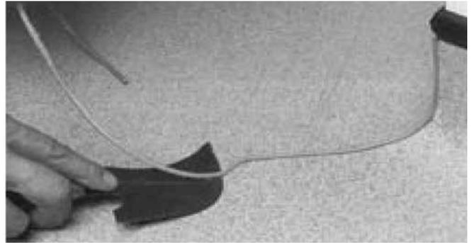
2. Allow the weldrod to cool completely, then trim surplus with the spatula. Chamfer off the external mitre with the square router blade.
