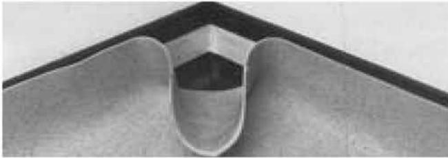
1. Once the main flooring is laid and adhered, push the flooring into the internal angle as far as possible. Make a cut from the base out to the top of the flooring in line with the mitre.
