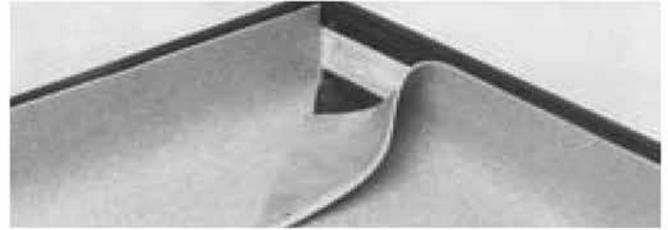
2. Fold in one side of the mitre and carefully cut off the surplus material. This completes the first part of the mitre.
