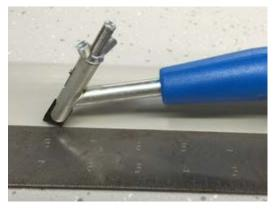
10. Once adhesive has cured, rout out seam for welding flooring material to shower transition trim with speed groover (AST SPEED).
