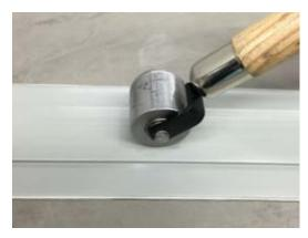
7. Roll shower transition trim firmly into the adhesive with a seam roller (AST RSH). Wipe away any excessive adhesive. Allow adhesive to cure.
