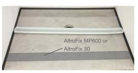
5. Apply AltroFix MP600 adhesive within the pencil lines and onto the cove former. Alternatively, AltroFix 30 adhesive can be used.
