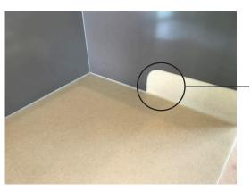
Finish by applying tamper-resistant security sealant where panel meets the floor. Cutout of wall to show pencil coved floor installed up and behind Altro Whiterock wall cladding for instructional purpose only.
