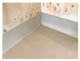
Heat weld the inside and outside corners in flooring before installing Altro Whiterock panels.
