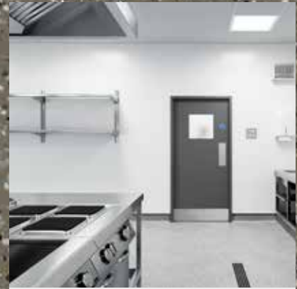
Fire performance: hygienic wall coverings to Class B-s3 d0, hygienic doorsets to FD60
