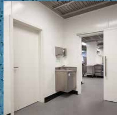
Wall fire resistance to Class 0; doors to FD60
