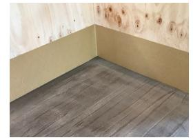
1A. Install contact tape for coving and spread adhesive on floor, note that there is no cove former used.
