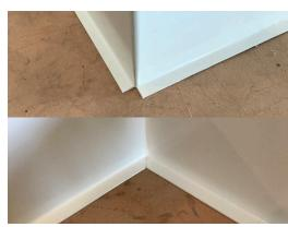
For internal corners, cut the rebate before bending. External corners require you to cut and mitre the rebate before bending.
