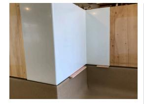
Make your inside and outside bends then install the corner panels. You will have to heat the face of the Altro Whiterock for certain bends being careful not touch the panel to the white insulating stones. Remove the protective film from the surface of the Altro Whiterock first.
