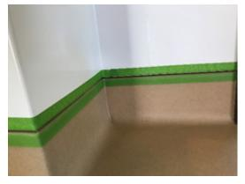
9. Tape off the rebate and apply tamper-resistant security sealant.
