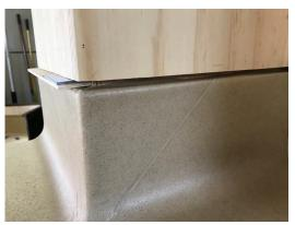
4. Once the material is heat welded, trim and tuck it into the rebate.
