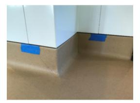
When heat welding the walls, place several layers of tape to prevent burning the floor. Once welded, trim any excess. When hanging straight walls, scribe and cut seams allowing for the appropriate gap for expansion and contraction (approx. 1/16") before you make your rebate bend (nothing larger than a 3d nail).
