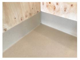
2. Heat weld the inside and outside corners in flooring before installing Altro Whiterock panels.
