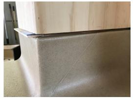
4. Once the material is heat welded, trim and tuck it into the rebate.
