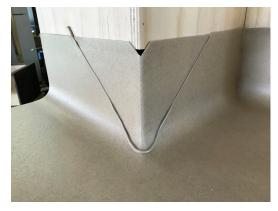
When installing outside corners, leave the rebate untucked to allow for heat welding.
