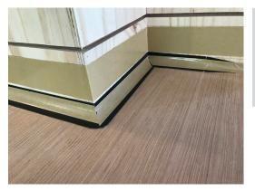
Apply contact tape on the wall as well as inside the rebate.
