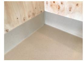
Heat weld the inside and outside corners in flooring before installing Altro Whiterock panels. When installing Altro Whiterock on an unleveled floor, you will have to scribe the panels to the floor.
