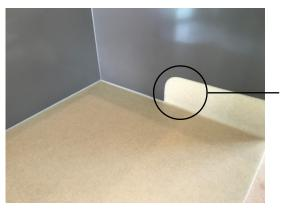
4. Finish by applying tamper-resistant security sealant where panel meets the floor.
