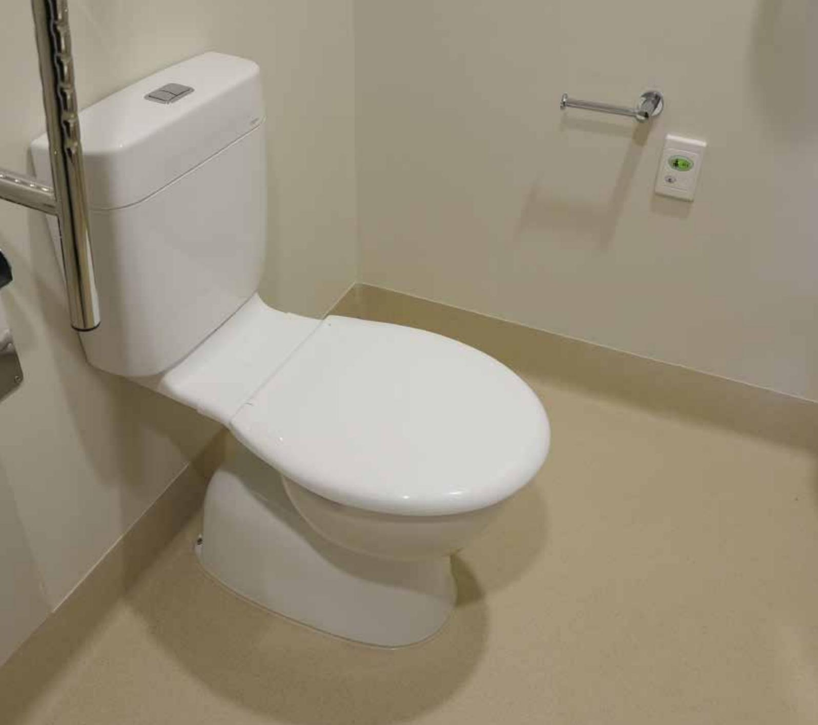
Altro Aquarius was used throughout the high care ensuites to ensure optimal safety in wet and dry, shoe and barefoot conditions. Achieving a pendulum test value of  $PTV \geq 50$  and Class B to DIN51097 for barefoot use, Altro Aquarius provides optimum lifetime sustained slip-resistance in wet and dry environments. It's a 2mm safety floor that has been extensively tested on a variety of shoe types to ensure top performance in a host of environments
