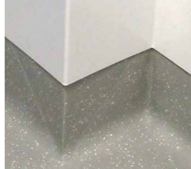
Overlap floor to wall transition
