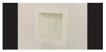
After the Installation is complete, the edges of the recessed shelf must be sealed with sanitary sealant to prevent water ingress.
