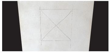
Use a datum line or other reference lines to determine the location on the wall substrate where the Altro Whiterock recessed shelf A900 will be installed. Transfer these measurements to the Tegulis panel and cut the panel opening approximately 10  $\frac{1}{8}$ " x 10  $\frac{1}{8}$ " for the 10" x 10" recessed body to fit into the cut out with ease.
