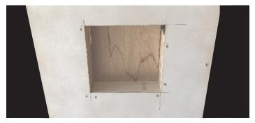
Adequate support must be within the wall substrate to support the recessed shelf and weight of its contents.
