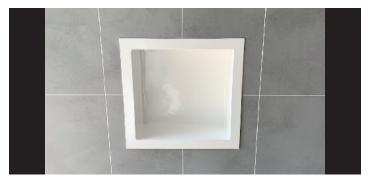
Apply AltroFix  $^{\text{TM}}$  MP600 to the back side of the flange. Install the recessed shelf into previously installed Altro Tegulis panel. Roll flange to ensure proper adhesive bond.
