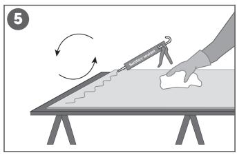
5. Clean the back of the panels to remove dust and contaminants. Apply Altro sanitary sealant on the back of the panel where it will overlap the existing coved flooring.
