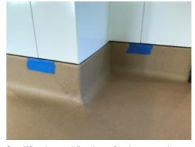
8. When heat welding the walls, place several layers of tape to prevent burning the floor. Once welded, trim any excess.
