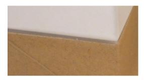
This is a detail that you might find in behavioral mental health installations, where a safe tamper-resistant joint detail is crucial, as well as installations where end-users may want to replace flooring in the future without damaging the wall system.
