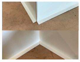
For internal corners, cut the rebate before bending. External corners require you to cut and miter the rebate before bending.
