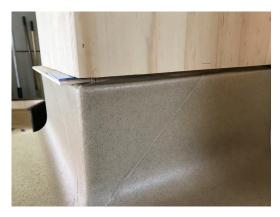
Once the material is heat welded, trim and tuck it into the rebate.
