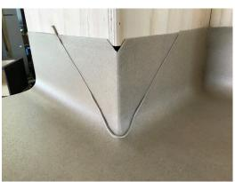
When installing outside corners, leave the rebate untucked to allow for heat welding.
