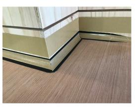
Apply contact tape on the wall as well as inside the rebate.
