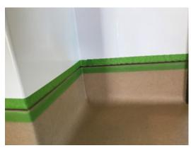
Tape off the rebate and apply tamper-resistant security sealant.
