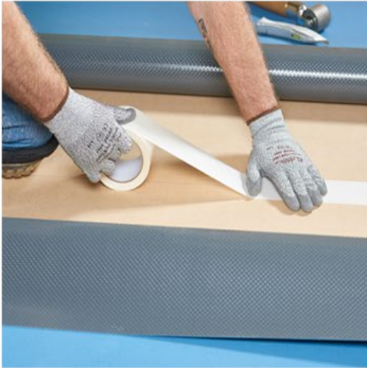
Tape at perimeter + seams
