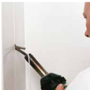
Altro Whiterock Welded joint
